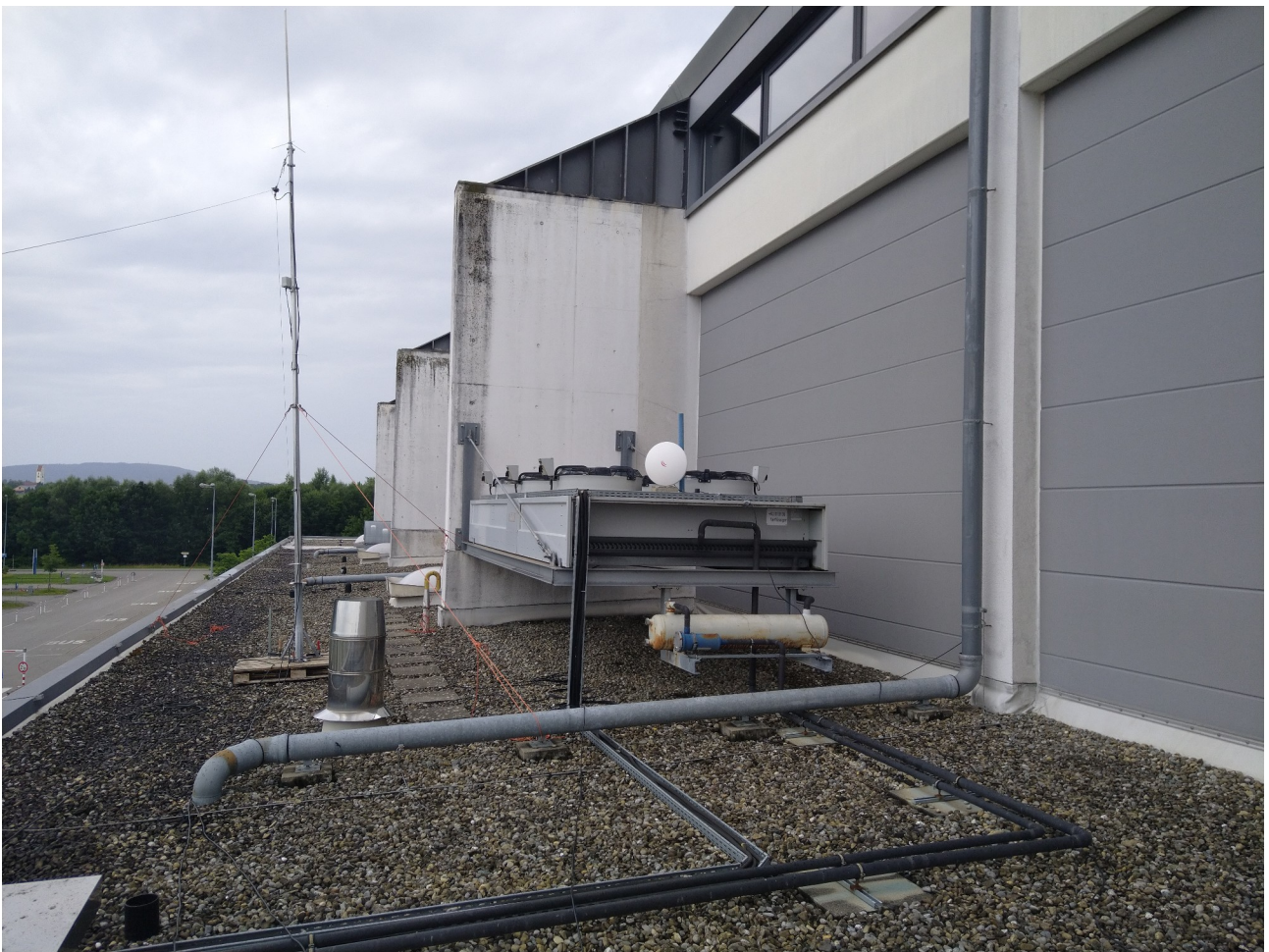
HAMNET connection of hall A1 via 5 GHz dish (center of picture on the air conditioning system)
